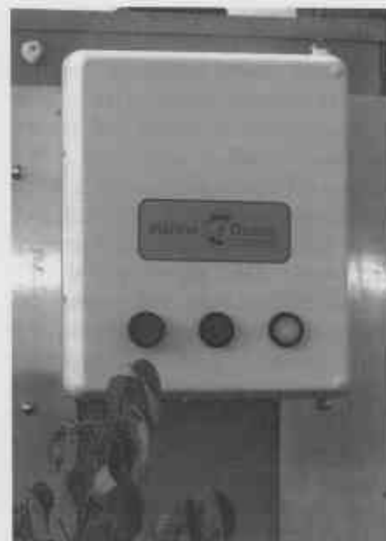
The ground fault monitor pictured here is used to monitor multiple connected boats from a central location.
